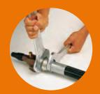
3 Screw on fully in a clockwise direction using spanners and counter spanners.
